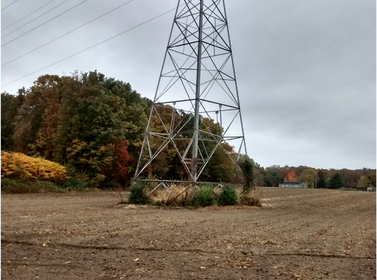
Figure 8: This agricultural span in Buena Vista Township is maintained by the landowner, not the utility. As a result, this span was not reported as being “managed” by the utility in the past six years.
